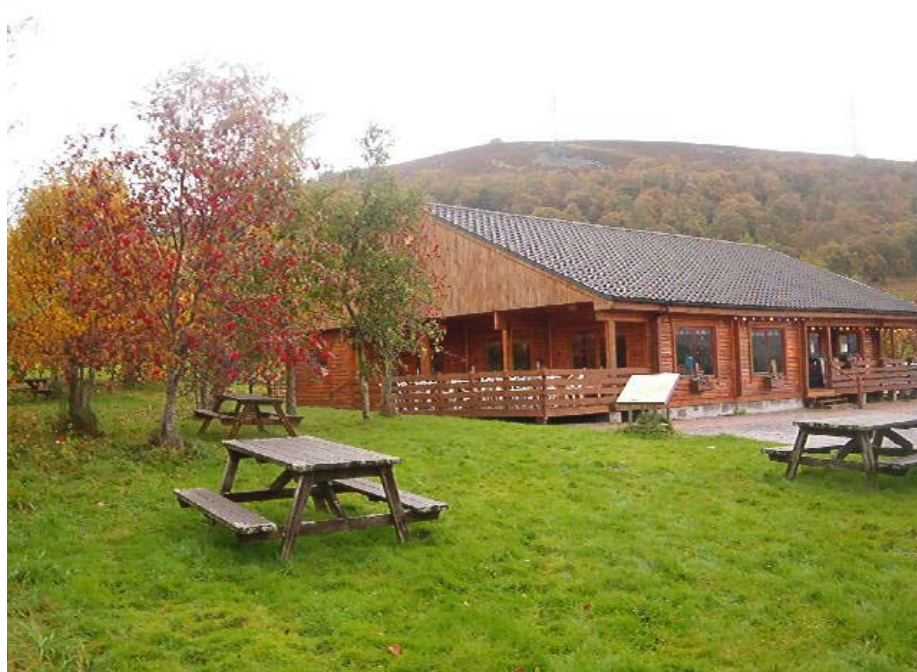
Fig. 3. Goodbrand & Ross Viewed from West Side
